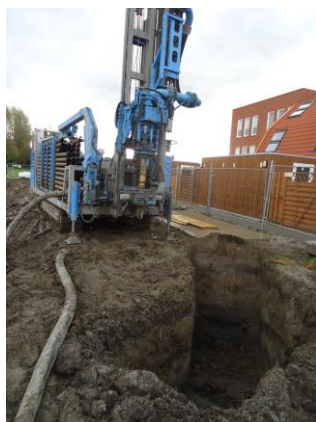
Positionering boorwagen locatie boring
